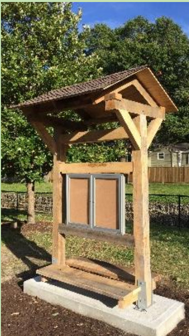
A timber-frame kiosk, installed at the tree-planting diversity demonstration site at Porter Park in Prairie Village.
